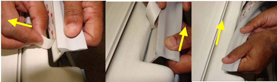
Remove outer liner of the adhered VHB tape for short distance as shown
