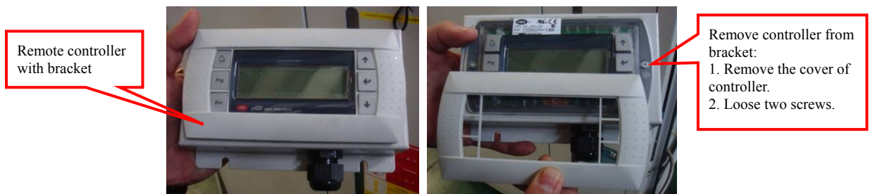
Fig.- 20 Remove remote controller from bracket
