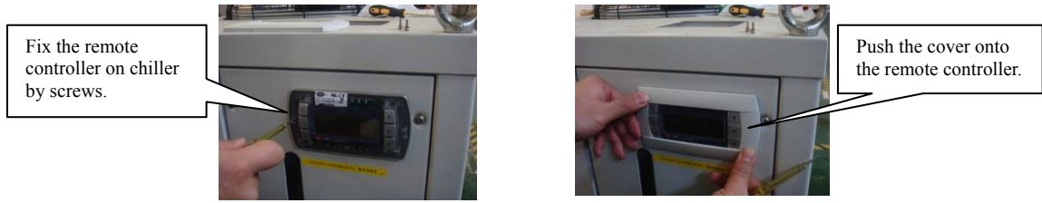
Fig.- 22 Fix remote controller on chiller
