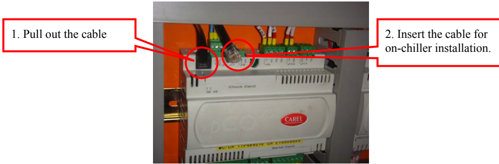
Fig.- 18 Remote controller cable connecting with controller
