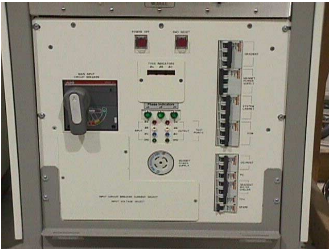
BREAKER LOCATION- PHOENIX PDU ILLUSTRATION 8-9
