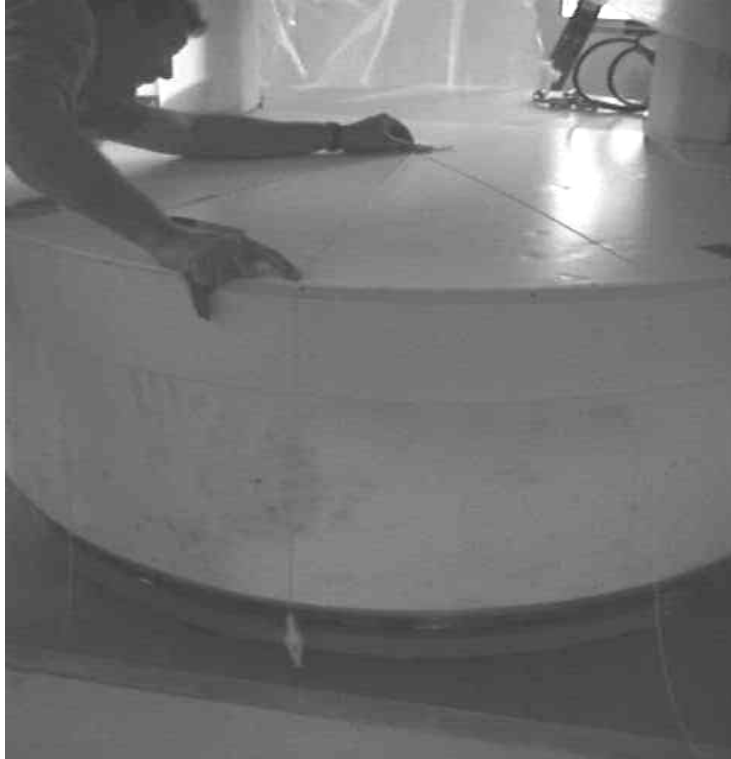
TRANSFERRING MARKS TO FLOOR ILLUSTRATION 4-11
