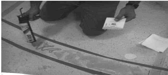
GLUING THE WEARPLATE/RACE TO THE FLOOR ILLUSTRATION 4-3
