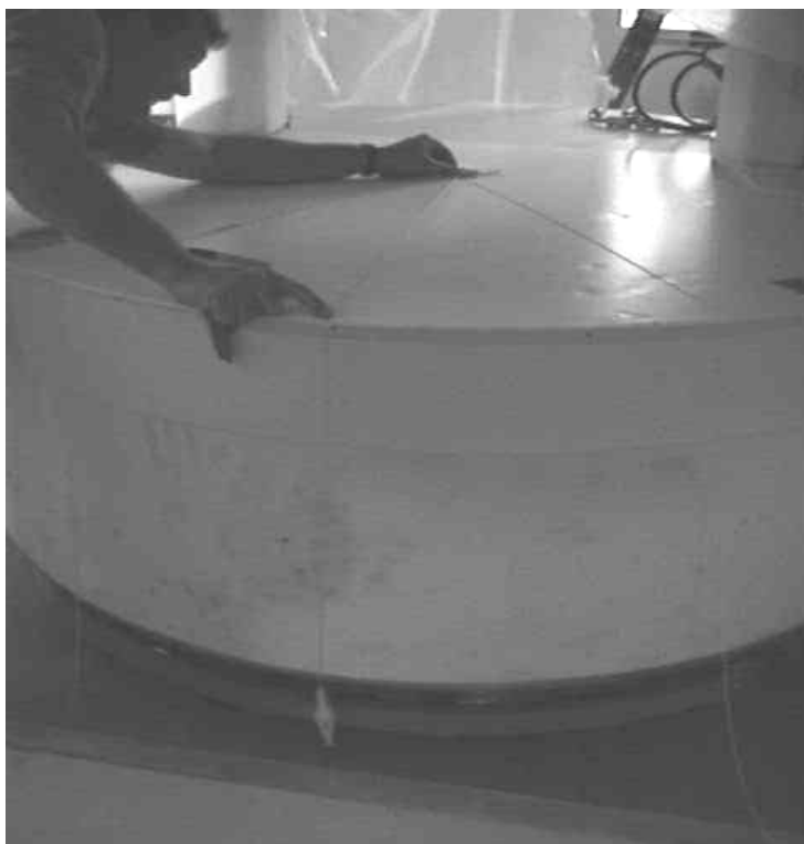
TRANSFERING MARKS TO FLOOR
