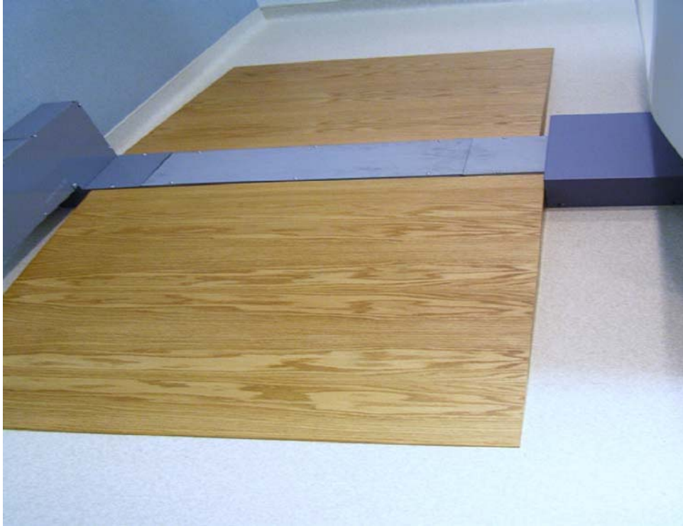
Figure 1-77 OSHA Ramp Example
