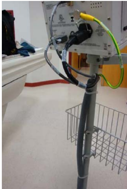
Figure 2-38 Cables Strain Relieved to Stand
