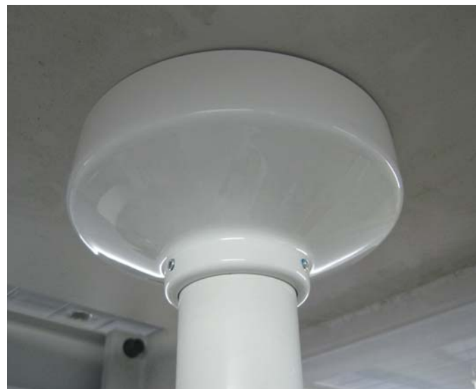
Figure 2-10 Pedestal Cover Installation
