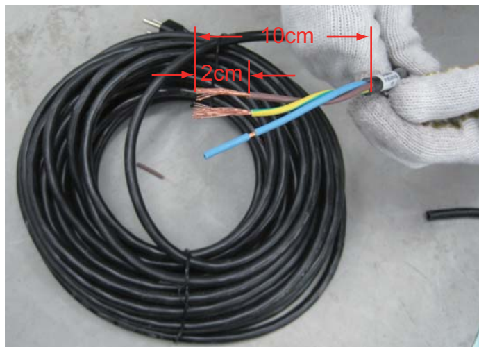
Figure 2-17 Remove the Scarfskin of Power Cable
