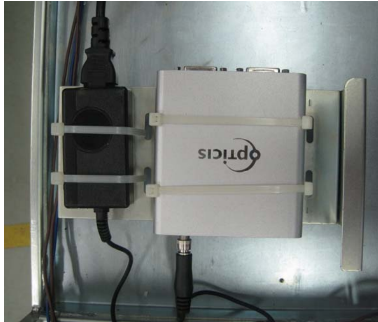
Figure 2-45 Attach Adapter and Splitter
