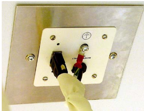
Figure 2-15 Finished Ceiling Plate
