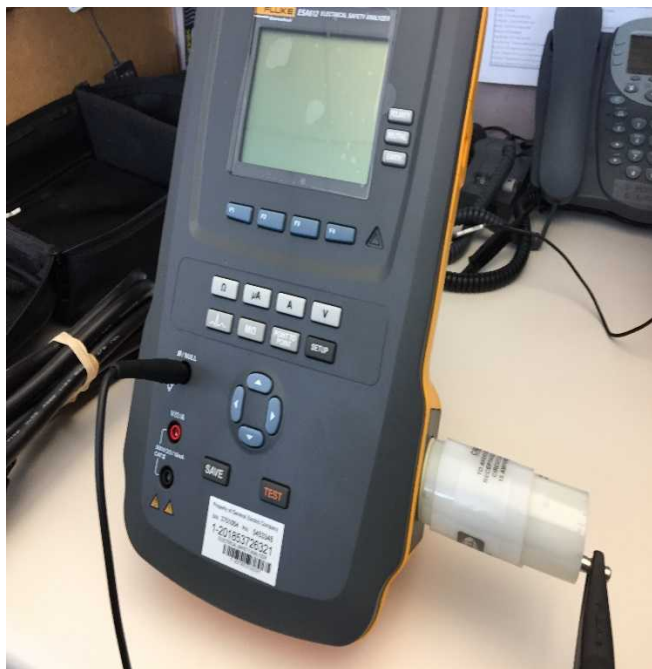
Illustration 6. Zeroing out Ground Wire Resistance when using the 15A to 20A Adaptor
