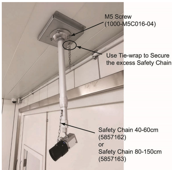
Figure 3-10 Example of safety chain for pipe bracket
