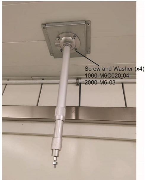
Figure 3-5 Extendable pipe installation
