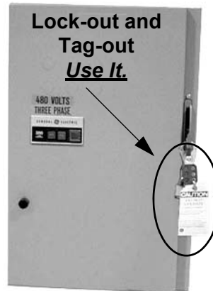
Figure 1-1 Sample PDB Breaker
