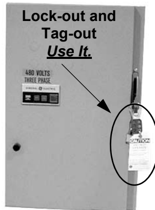
Figure 2-1 Sample PDB Breaker
