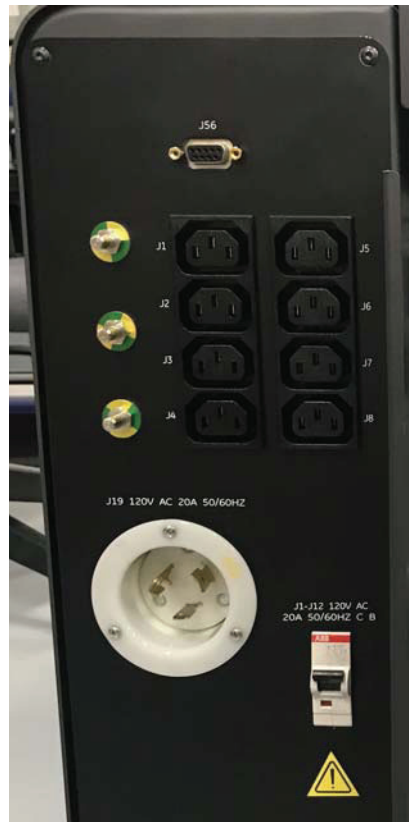
Figure 3-38 OpenOC AC Box Connections
