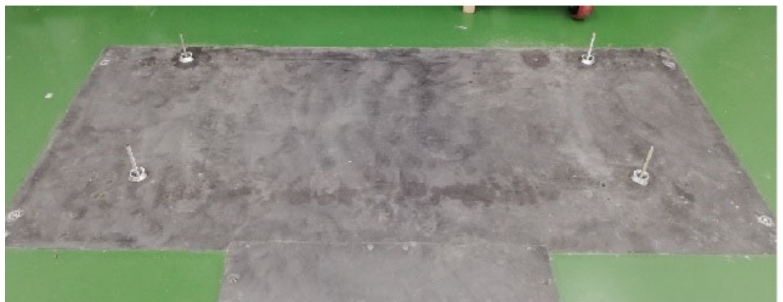
Figure 2-29 Gantry Anchor Bolts
