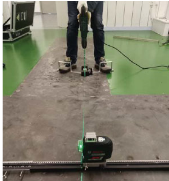
Figure 2-26 Drill Table Anchor Holes
