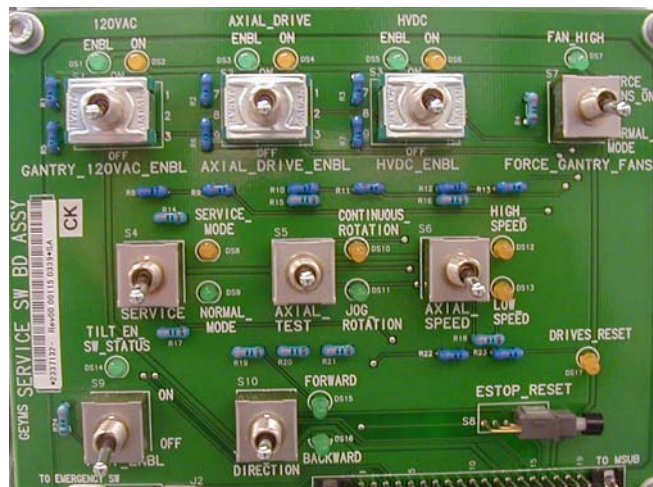
Figure 3-3 LightSpeed Gantry Service Switches
