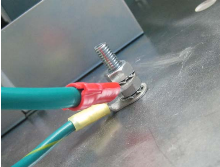
Figure 2-26 Ground Cable Connection
