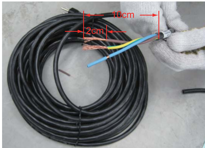
Figure 2-17 Remove the Scarfskin of Power Cable
