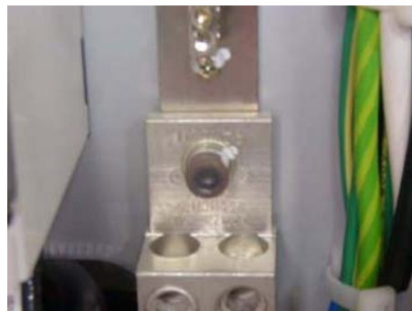
Figure 1-79 PDU System Ground Connection
