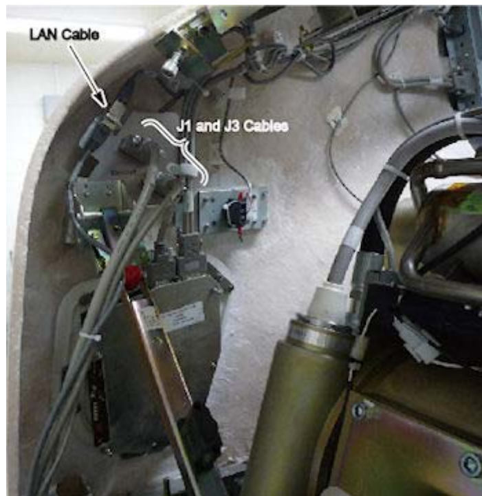
Figure A-19 Front Cover Cables
