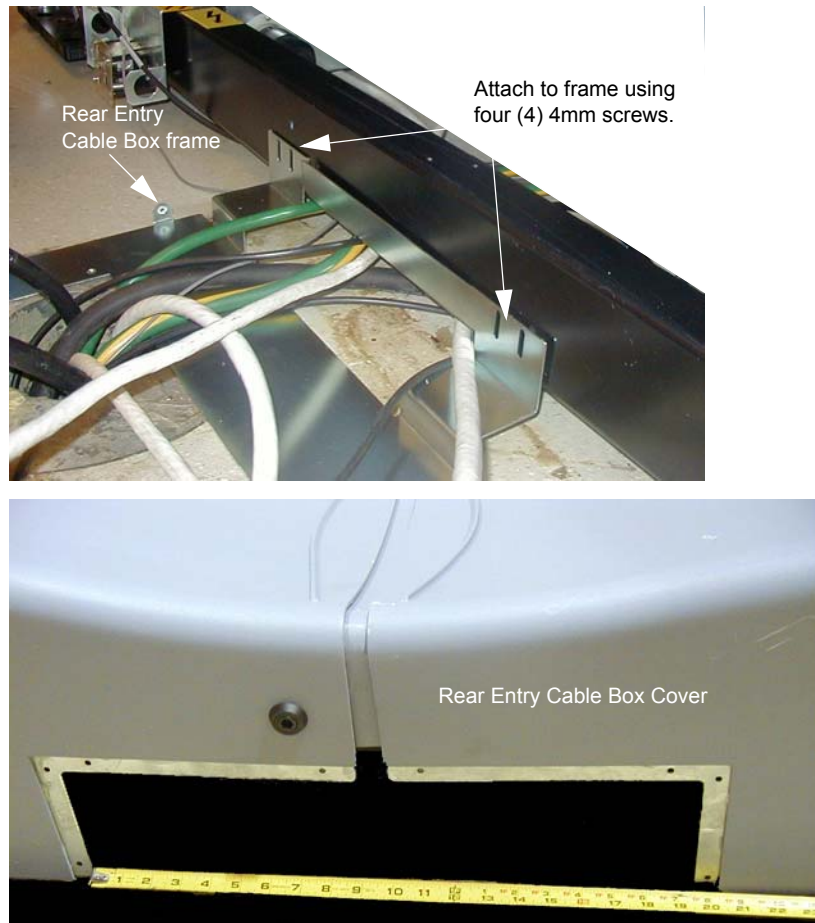
Figure 1-65 Rear Entry Cable Box
