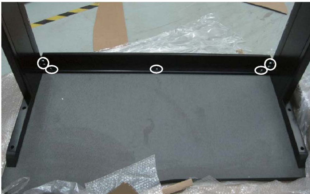
Figure D-3 Crossbar Installation
