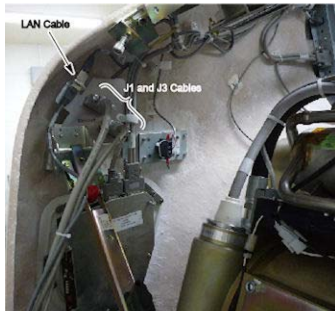
Figure A-14 Front Cover Cables
