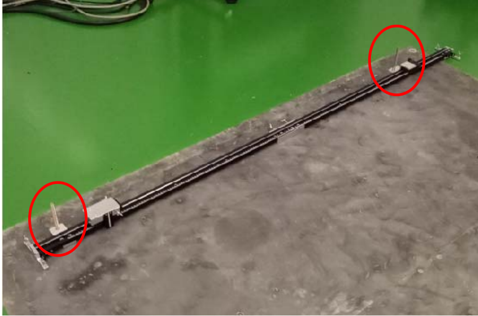
Figure 2-14 Sliding Rail Installation (example)
