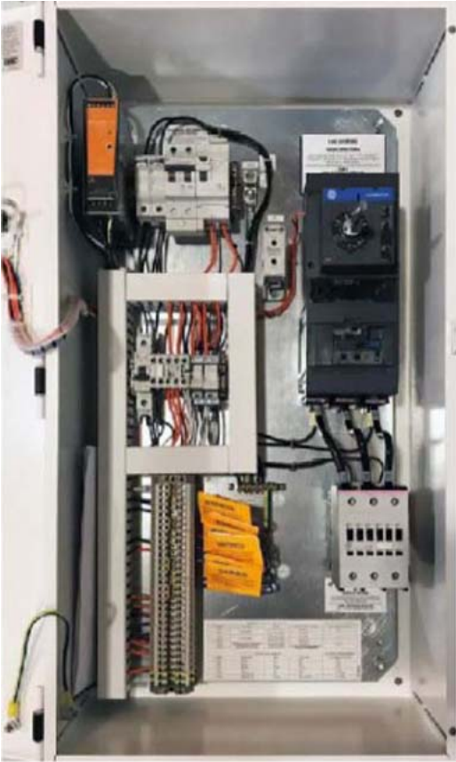
Figure 13-10 Primary Power Disconnect (A1/MDP- E4502AB/E4502AC)
