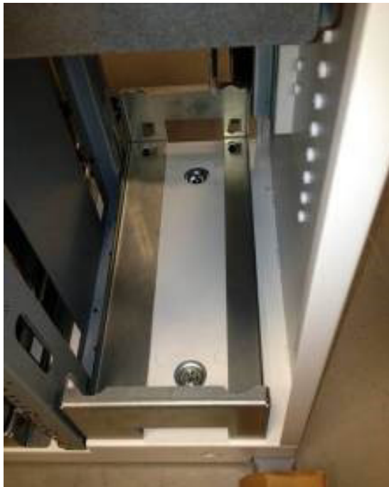
Figure 2-20 Install Service Platform
