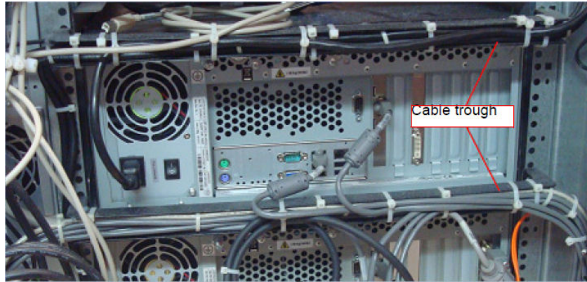
Figure 2-3 Remove Plates and Cables
