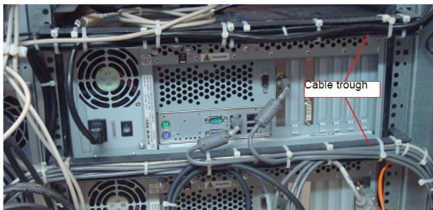
Figure 2-20 Install New Cable Trough
