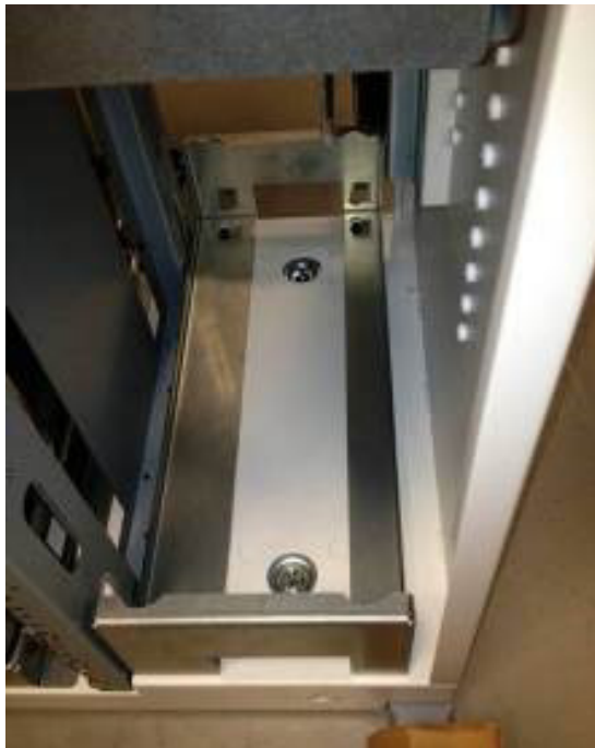
Figure 2-20 Install Service Platform
