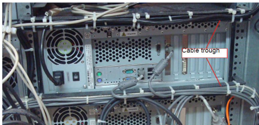
Figure 2-20 Install New Cable Trough
