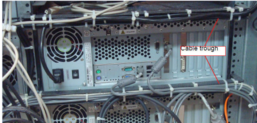
Figure 2-3 Remove Plates and Cables
