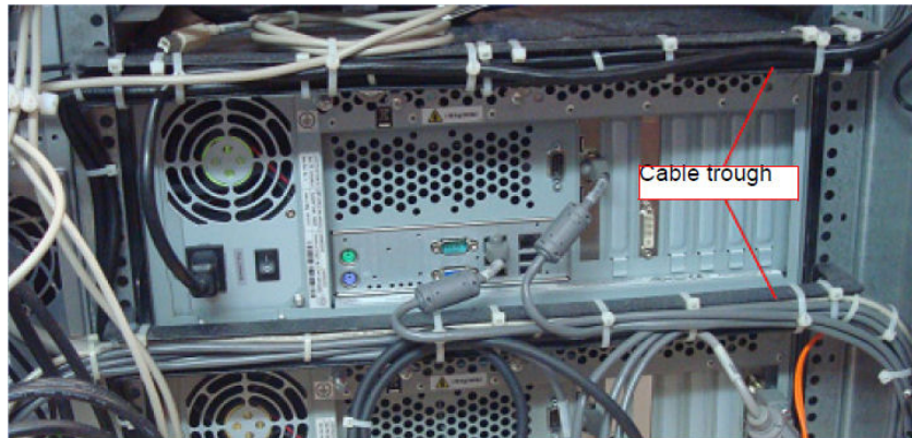
Figure 2-3 Remove Plates and Cables
