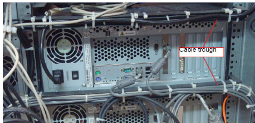
Figure 2-22 Install New Cable Trough
