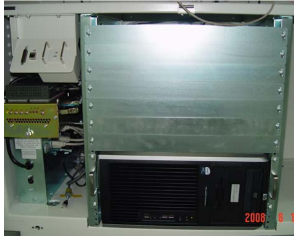
Figure 2-1 Metal plates installed at front of console
