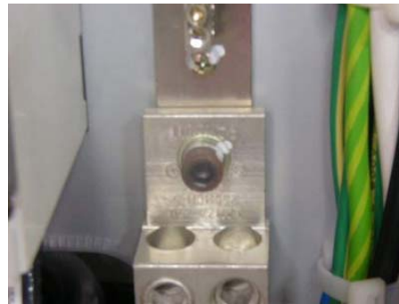
Figure 2-79 PDU System Ground Connection
