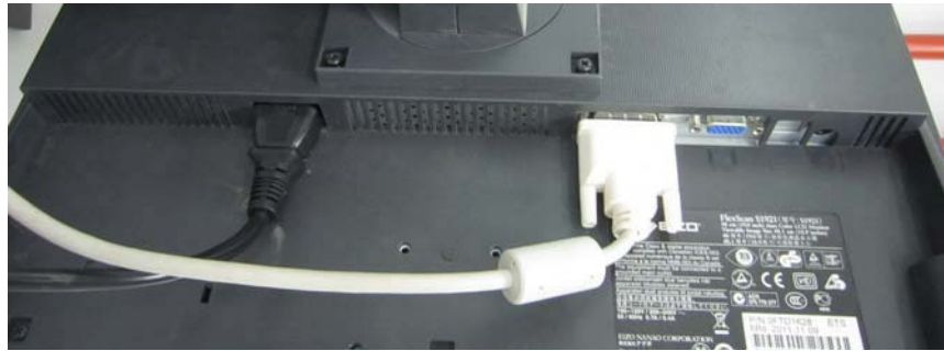
Figure 2-39 Video Cable and Power Cable
