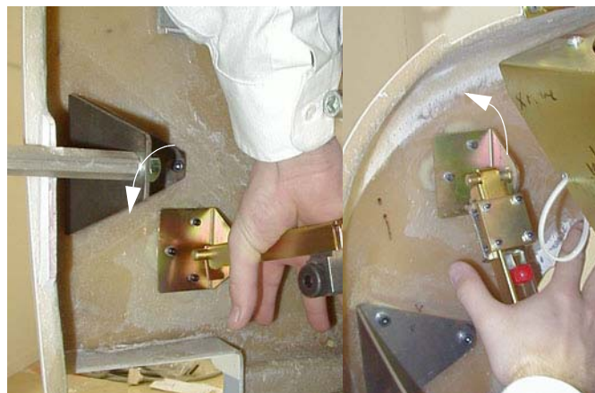
Figure A-21 Locking the cover brackets into place
